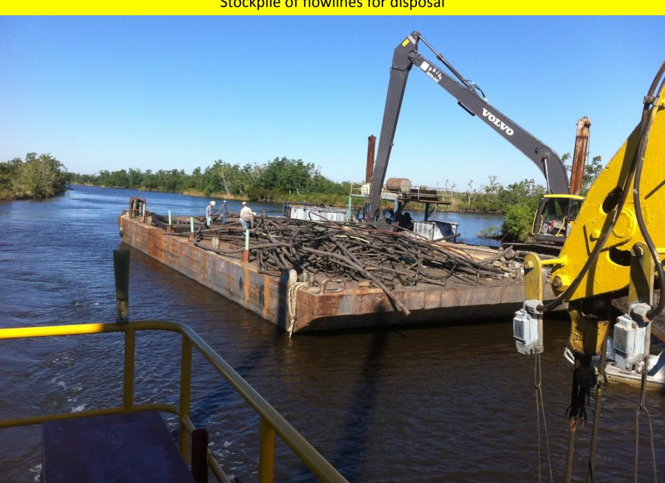
Cutting flowlines into manageable size sections
