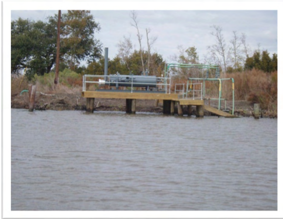
PC150030: Newly constructed platform with heater
