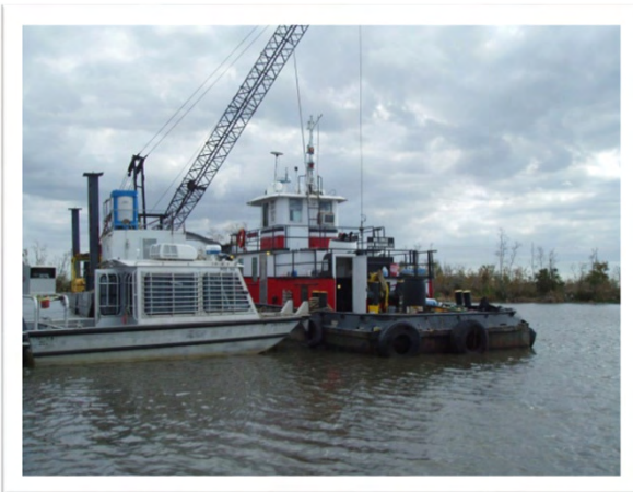
PC150040: Crane/barge/tug used for flowline/pipeline removal
