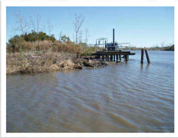
PC130002: Newly constructed platform with heater treater
