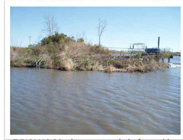
PC130003: Newly constructed platform with heater treater and flowlines
