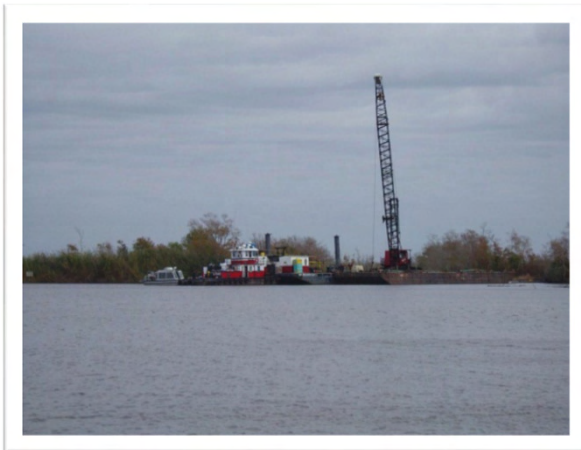
PC150032: Crane/barge/tug used for flowline pipe removal
