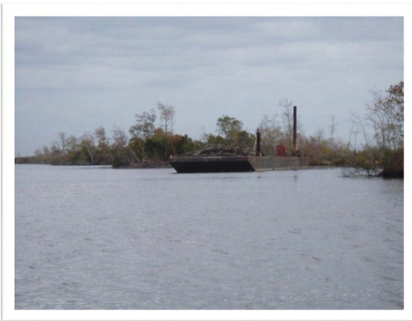
PC150028: Barge holding flowline and pipe removal debris
