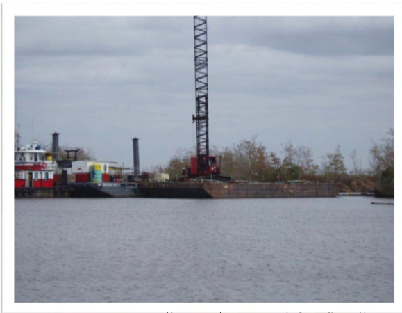
PC150036: Crane/barge/tug used for flowline pipeline removal
