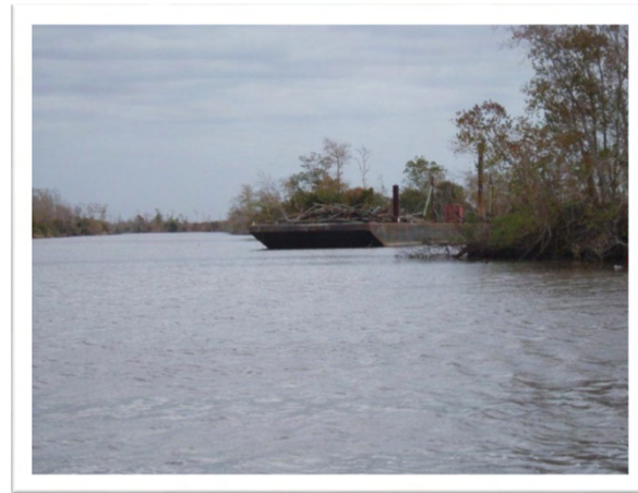
PC150027: Barge holding flowline and pipe removal debris
