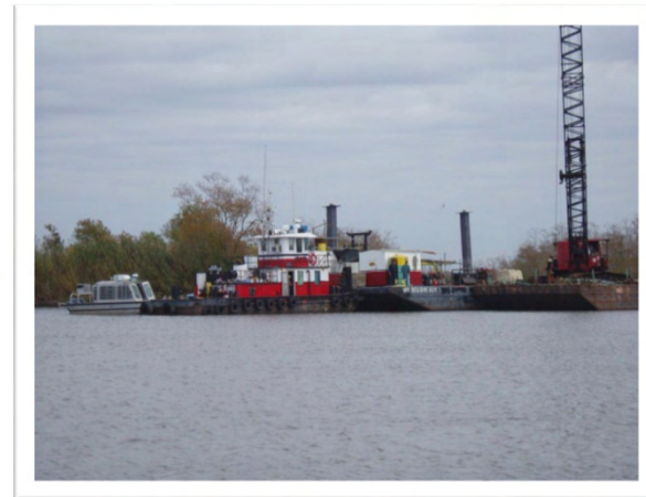
PC150037: Crane/barge/tug used for flowline pipeline removal
