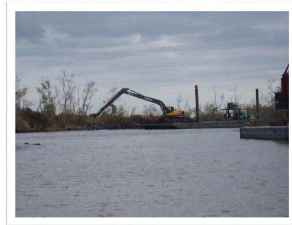
PC150041: Long stick on barge conducting flowline/pipeline removal
