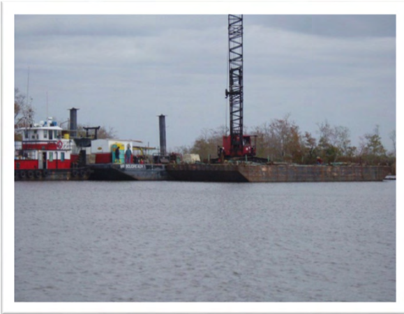
PC150038: Crane/barge/tug used for flowline pipeline removal
