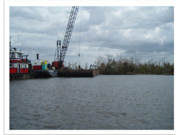
PC150039: Crane/barge/tug used for flowline/pipeline removal
