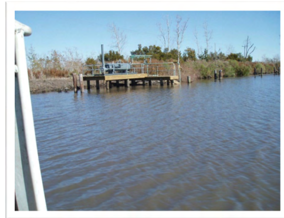
Newly constructed platform with heater treater
