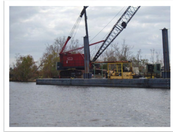
PC150043: Crane on barge conducting flowline/pipeline removal
