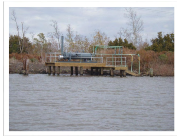
PC150029: Newly constructed platform with heater
