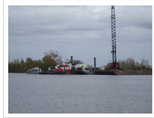
PC150035: Crane/barge/tug used for flowline pipeline removal
