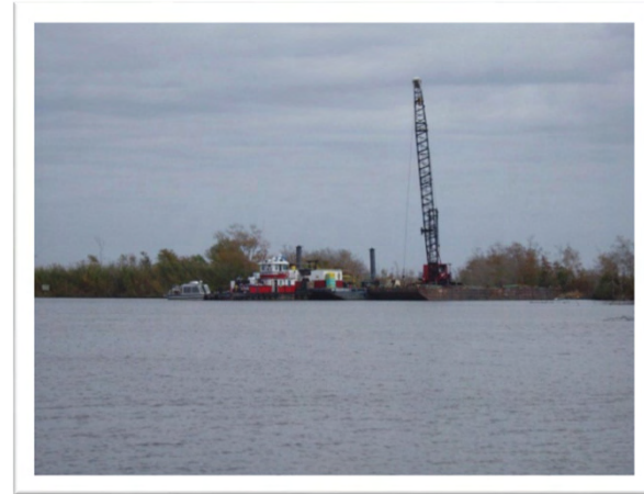
PC150031: Crane/barge/tug used for flowline pipe removal
