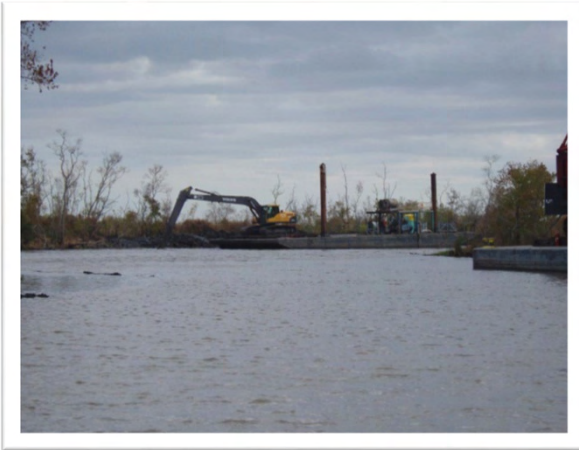
PC150042: Long stick on barge conducting flowline/pipeline removal
