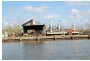
Main Operating Facility 110
