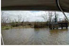
Due S of Facility 097
