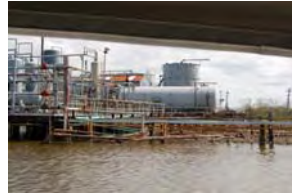
Facility S Bank 102
