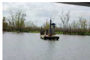
Well S Schooner E Facility 118
