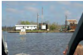
Facing N at Facility 101
