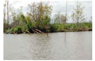
Flowlines S Schooner E Facility 115
