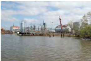
Facing N at Facility 099
