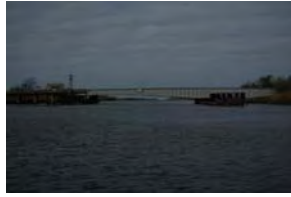
Schooner Bayou Canal Little Prairie Bridge 032
