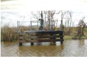
Due S of Facility 096
