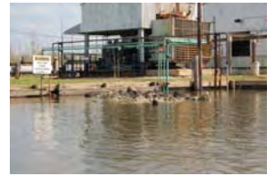
Soil at Facility 109
