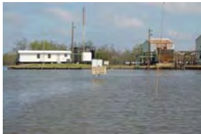
Facing N at Facility 100
