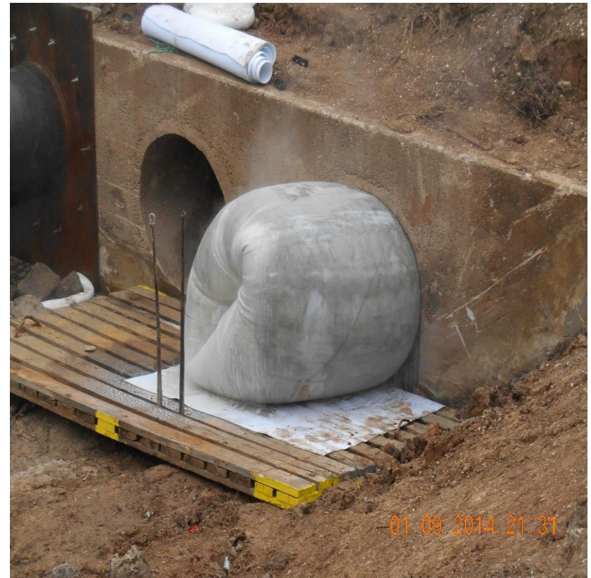
The dewatered site and a liner exiting the siphon
