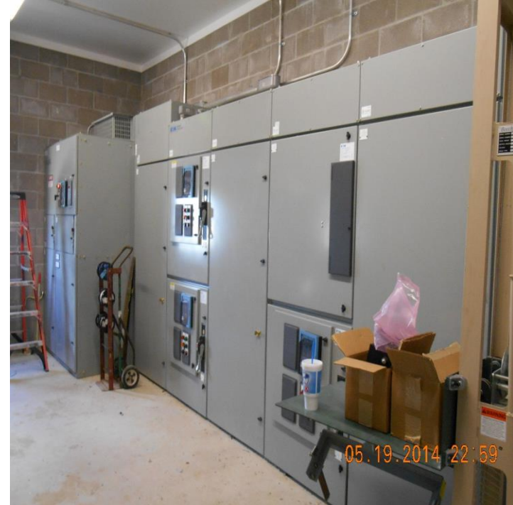
Switchgear Cabinets
