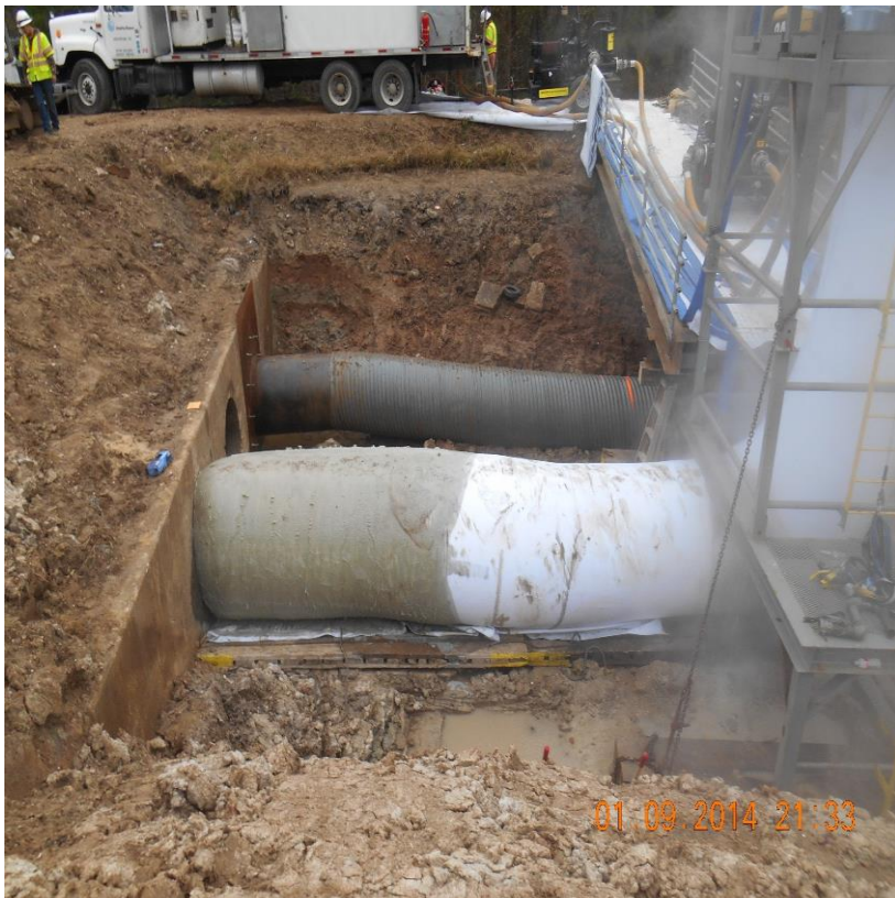
The dewatered site and a liner being installed
