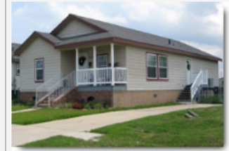
Brick veneer with traditional New Orleans circular vents. Elevation about 3 ft.
