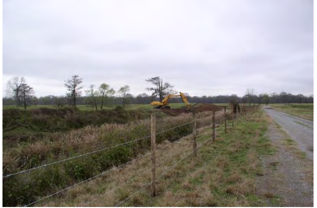
Decrease Non-Point Source - Channel Fencing
