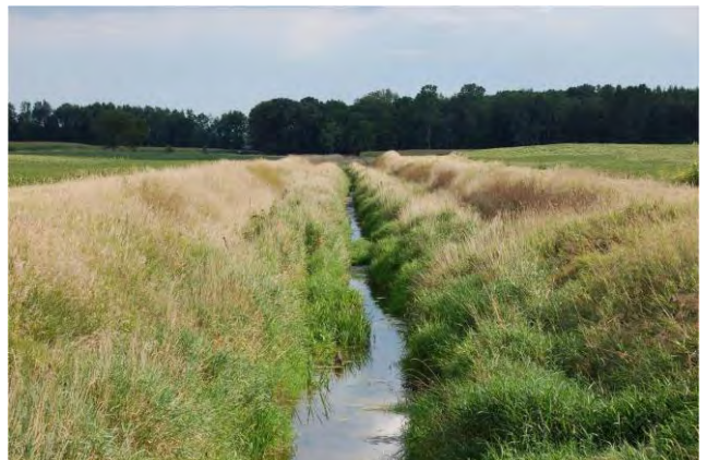
Increase Storage -Two-Stage Ditch
