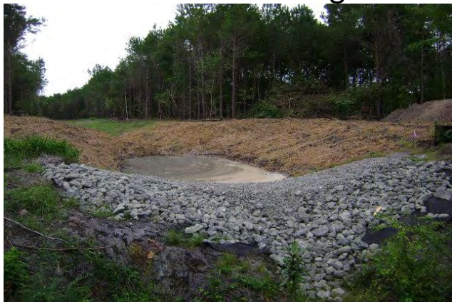
Flow Retardation -Rock Weir
