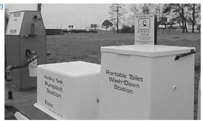
pumpout units and portable toilet washdown stations to properly and legally dispose of boat sewage (22). Without pumpouts and washdown stations, raw sewage could be released into marina basins or adjacent waters, degrading the most important areas of marina business.
