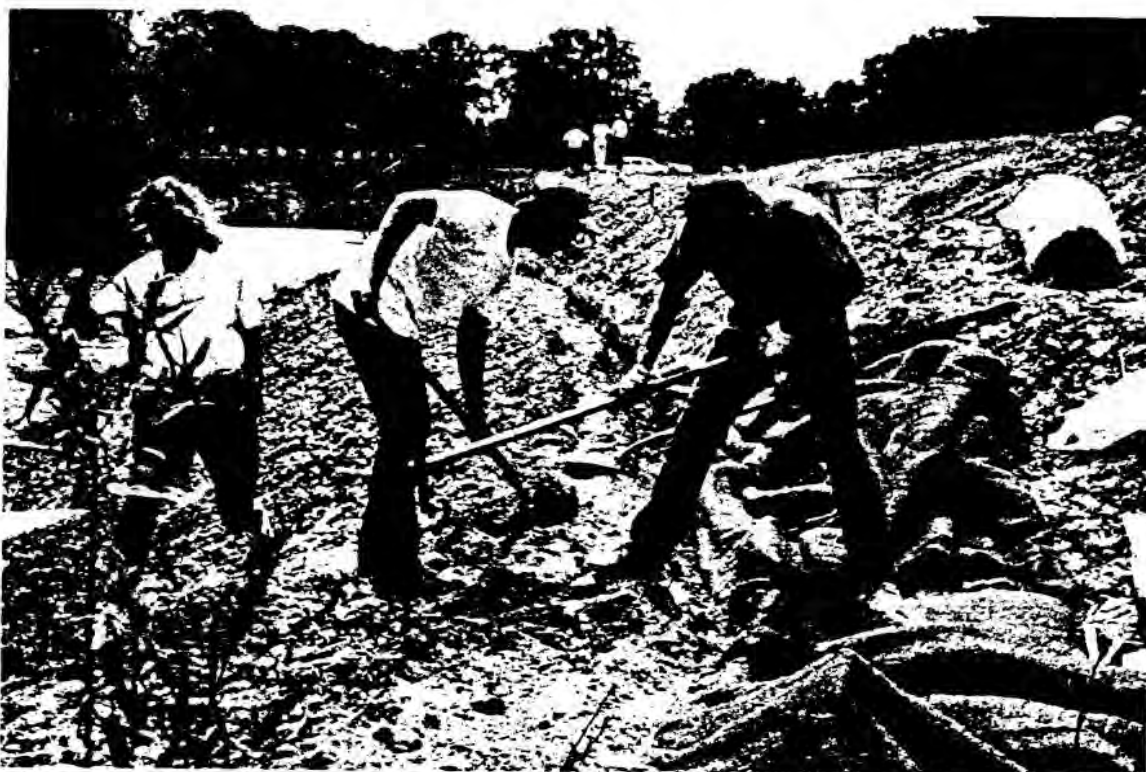
Figure 5. Geotextile cloth is stapled to the bank to protect seed and prevent erosion (pictured are personnel from the Soil Conservation Service's Plant Material Program).
