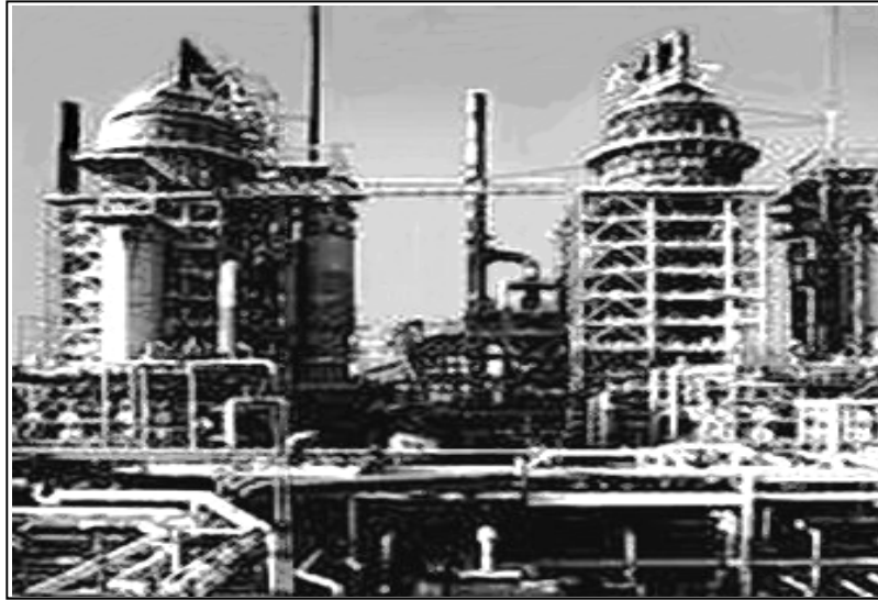
Exxon-Mobil Refinery - Baton Rouge
