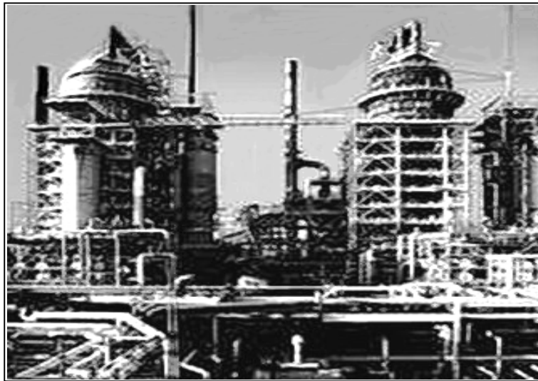
Exxon-Mobil Refinery - Baton Rouge
