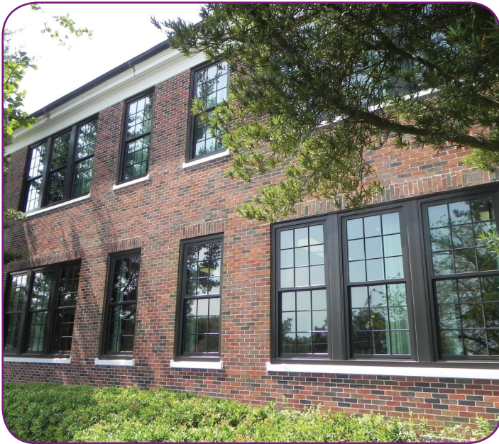
NICHOLLS STATE BUILDINGS - LEAD BY EXAMPLE WINDOW REPLACEMENT
