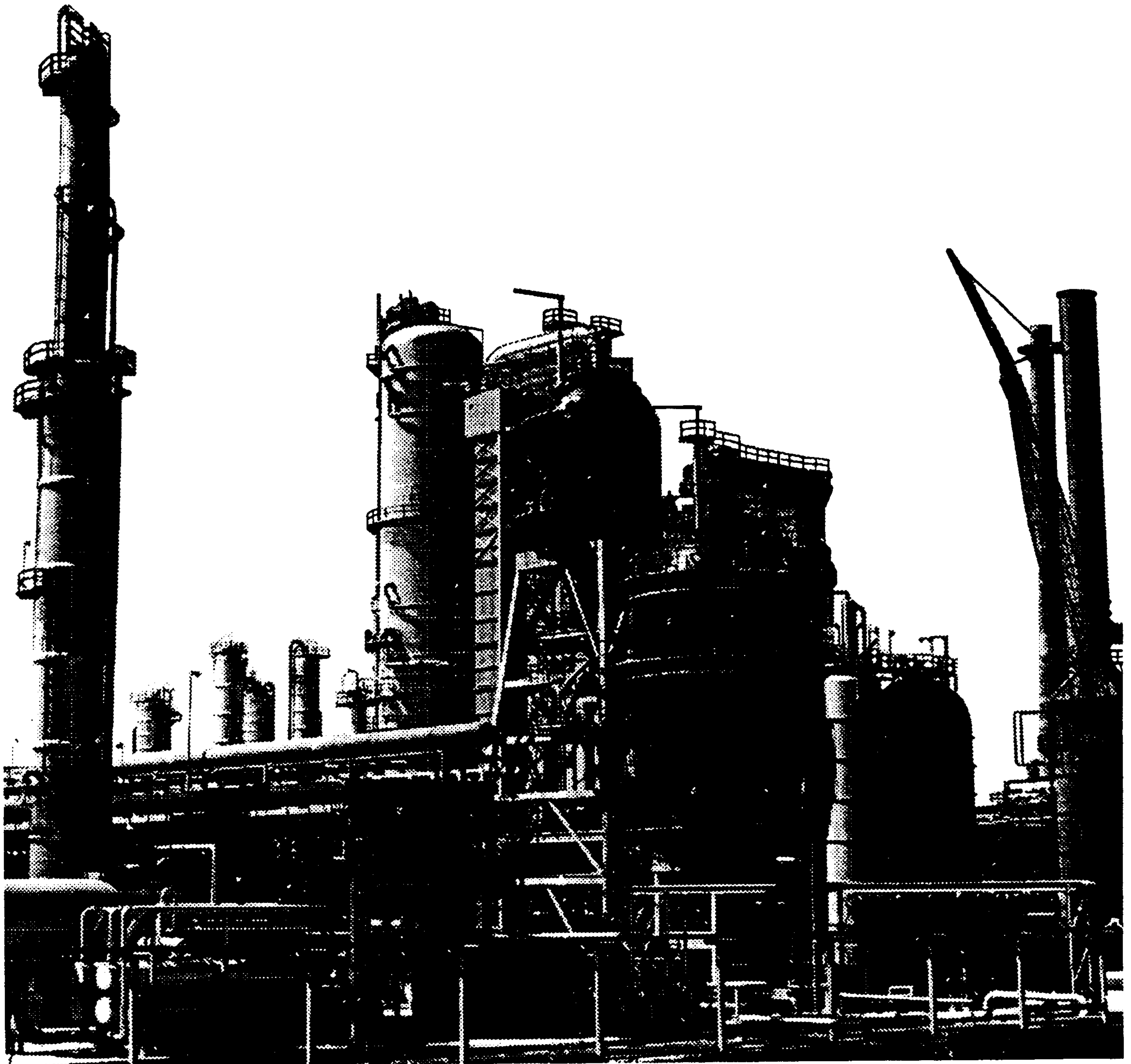
As part of the refining process, a catalytic cracking unit is used to increase the yield of gasoline from crude oil.
