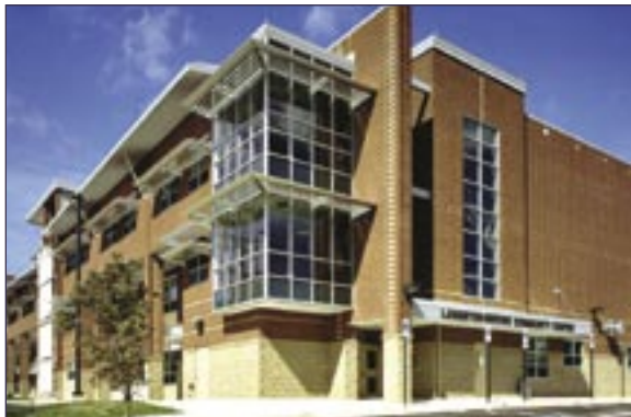
Shades on the southwestern windows of Langston High School in Arlington, Virginia, help maintain livable thermal conditions in the building, even when the power goes out.
