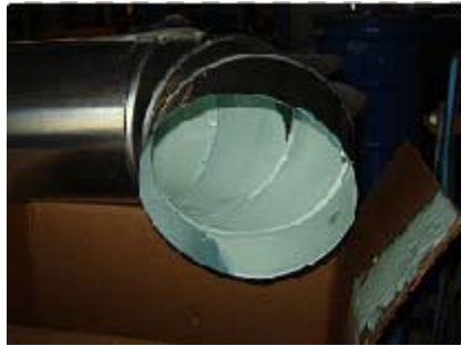
Figure 10-9. Elbow coated with polar seal primer
