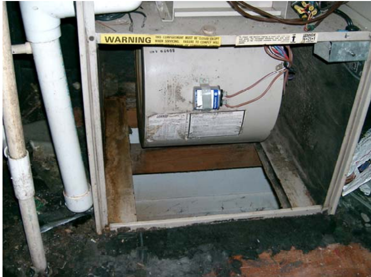
Figure 5-4. Placement of blockage to seal of the supply side.
