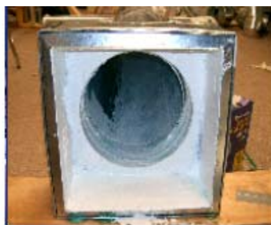
Figure 9-20 Sealant applied on the register
