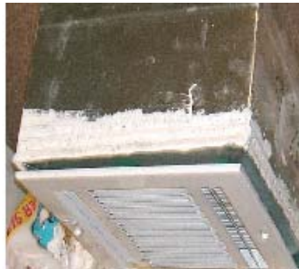
Figure 9-8. Sealant applied on the register boot
