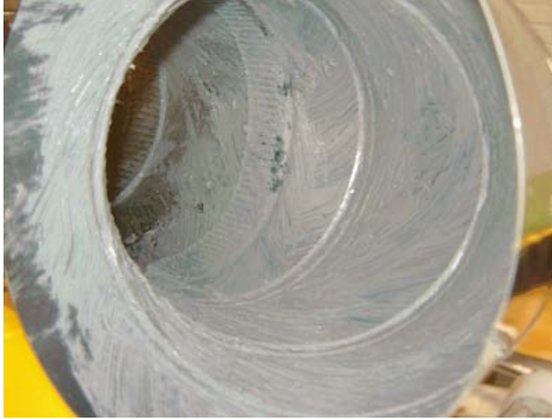
Figure 10-10. Photo of duct sealed with brush applied duct sealing mastic (good filling of cracks; crusting within 30 min, thus preventing flowing out of filled areas)
