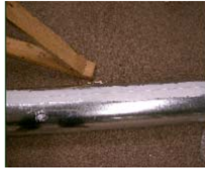
Figure 9-12. Sealant applied on the seam
