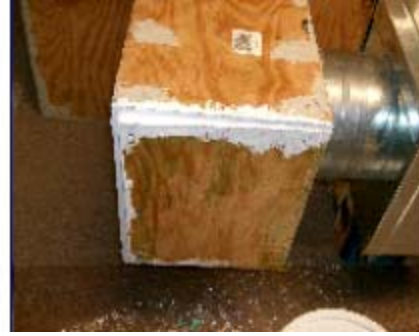
Figure 9-4. Sealant applied along the edges
