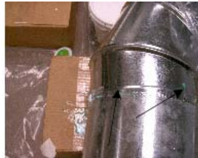
Figure 9-16. Flow of sealant to outside
