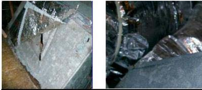
Figure 6-1. Common sources of supply duct leakage.
