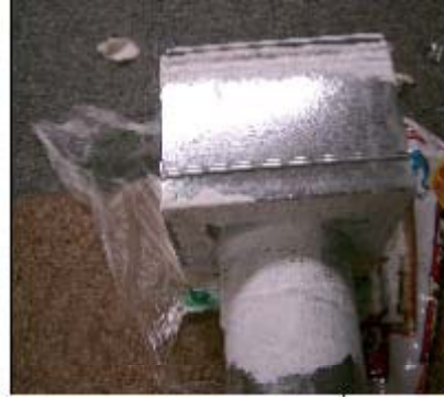
Figure 9-10. Sealant applied at joints with registers
