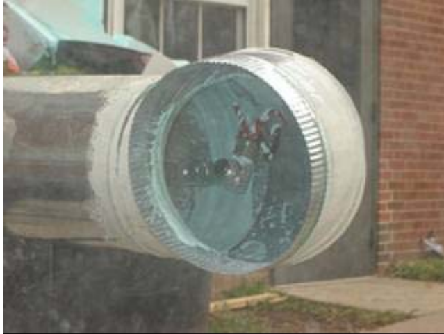
Figure 10-8. Primer being applied with 90° nozzle configuration
