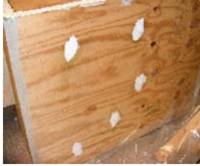
Figure 9-3. Sealant applied on drilled holes
