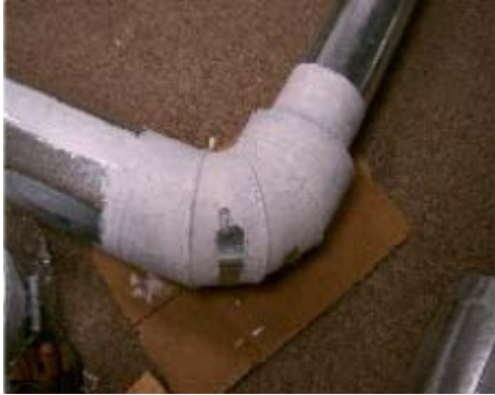
Figure 9-9. Sealant applied at joints with turns
