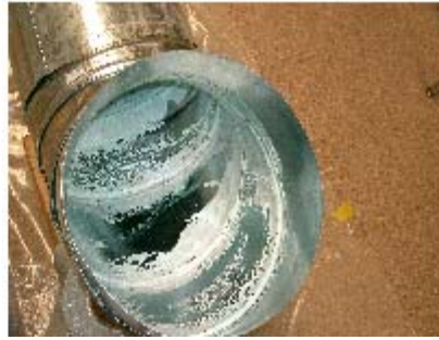
Figure 9-14. Sealant applied on turns/joints.
