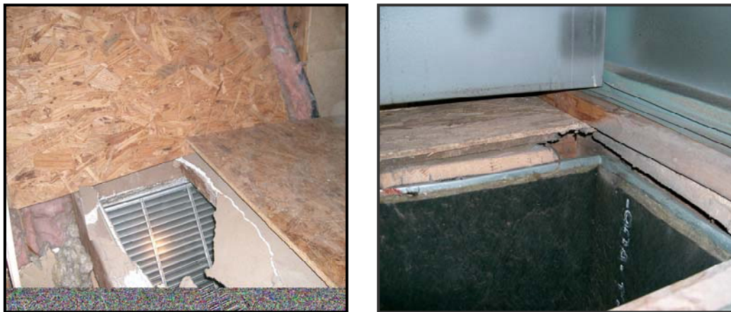
Figure 5-2. Common spots of return leaks.
