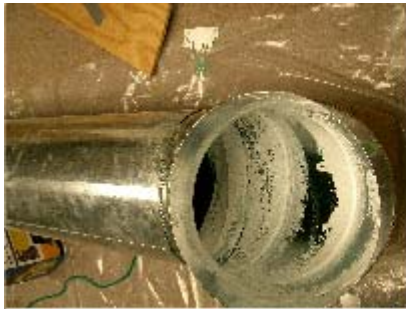
Figure 9-15. Sealant applied on turns/joints.
