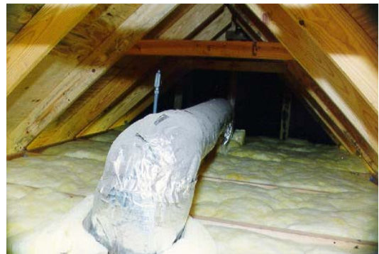
View of the attic in the fiberglass bldg.
