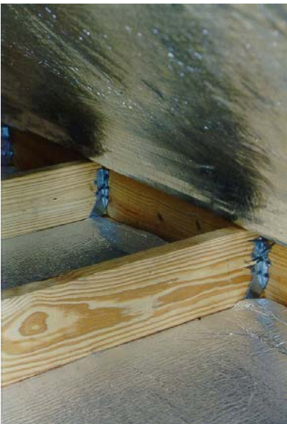
View of the attic in the radiant barrier bldg.
