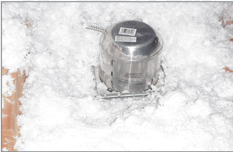
Sealed can (only air tight with an insert) – note holes in side where air can enter the home through the attic (attic temps in summer can be >140 degrees)
