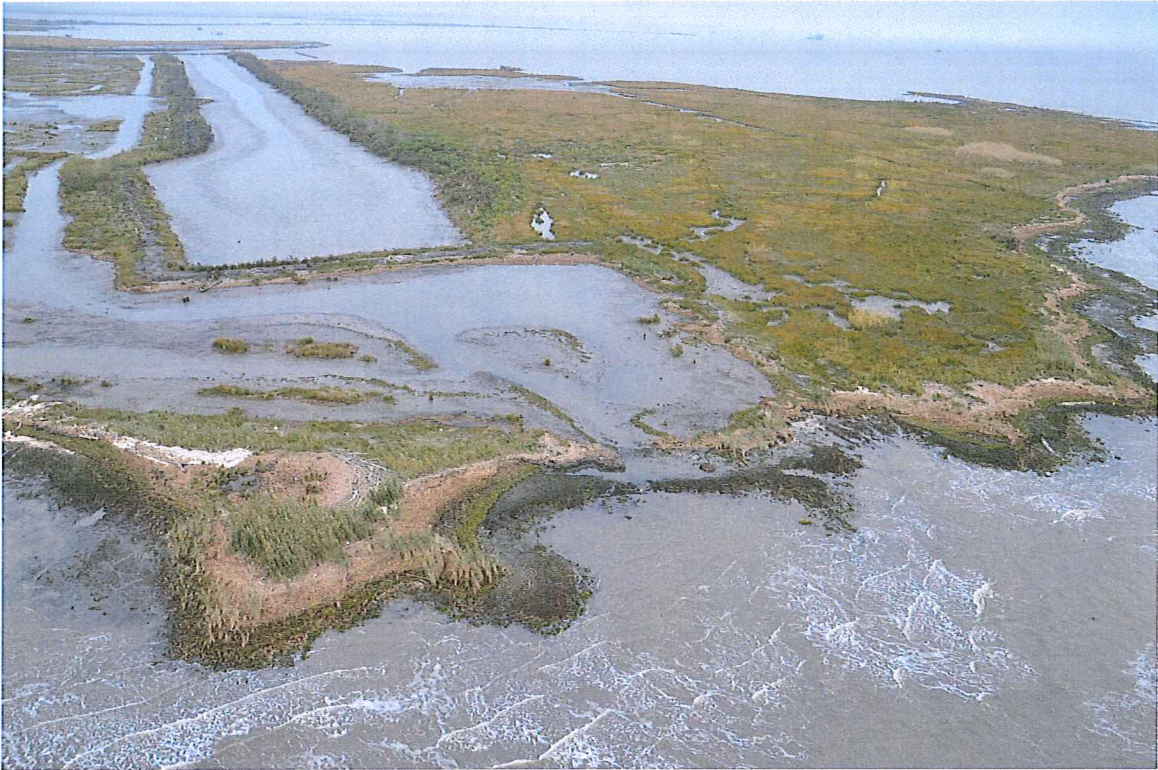
Figure 5. Bid Items 6, 7, and 8 - Shoreline Protection looking West (Date Taken 12-11-13)
