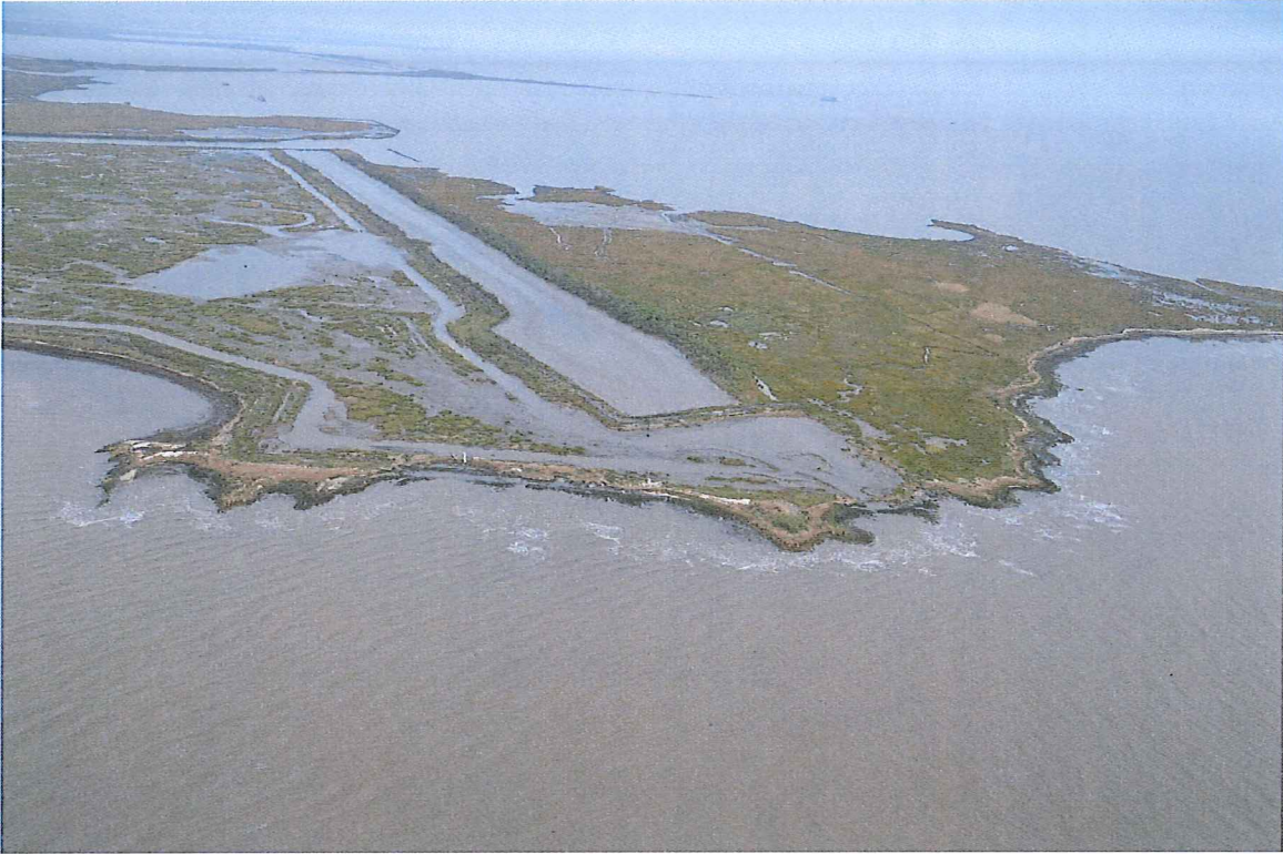
Figure 3. Bid Items 6, 7, and 8 - Shoreline Protection looking West (Date Taken 12-11-13)
