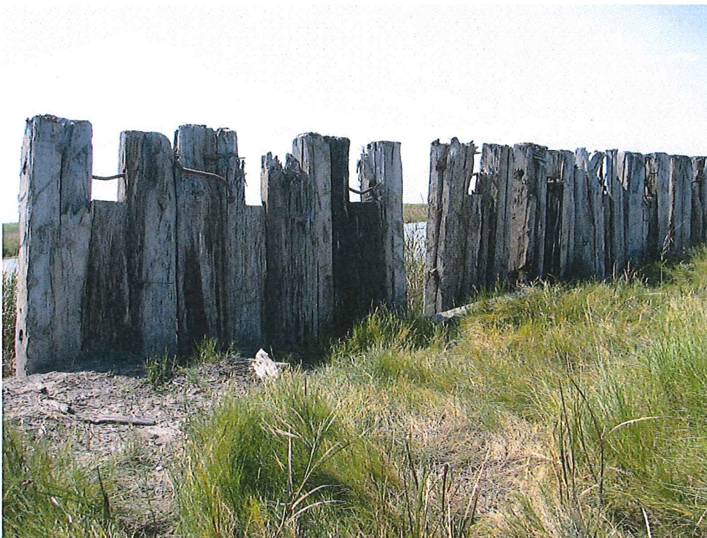
Figure 2. Bid Item 4 - Timber Mats (Date Taken 9-26-12)
