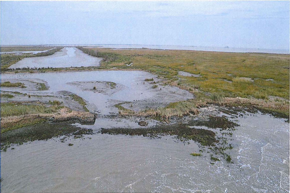
Figure 6. Bid Items 6, 7, and 8 - Shoreline Protection looking West (Date Taken 12-11-13)
